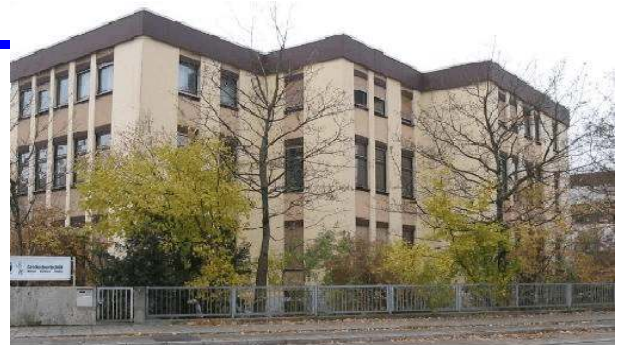
VAU Werkzeug's facility in Munich, Germany
